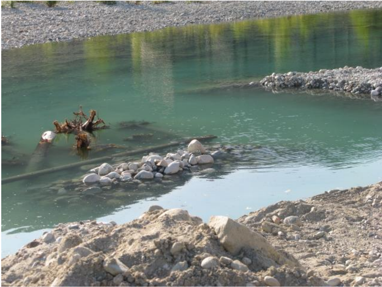
Backfilling a log-jam after being set into the water. September 2 nd , 2008.
