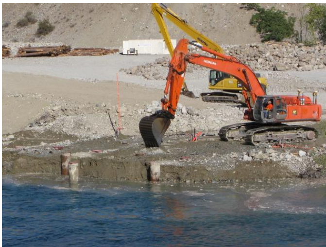
Removing the temporary earth berm from around the drilled piers. September 10 th , 2008.
