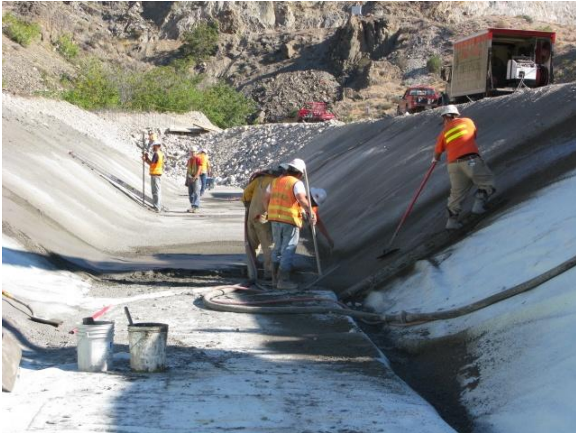
Shotcrete installation on top of conveyance canal liner. August 13 th , 2008.
