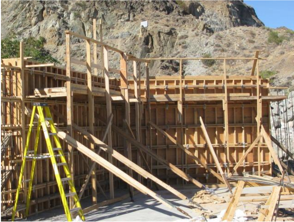
Wall forming for the outlet control structure. September 10 th , 2008.
