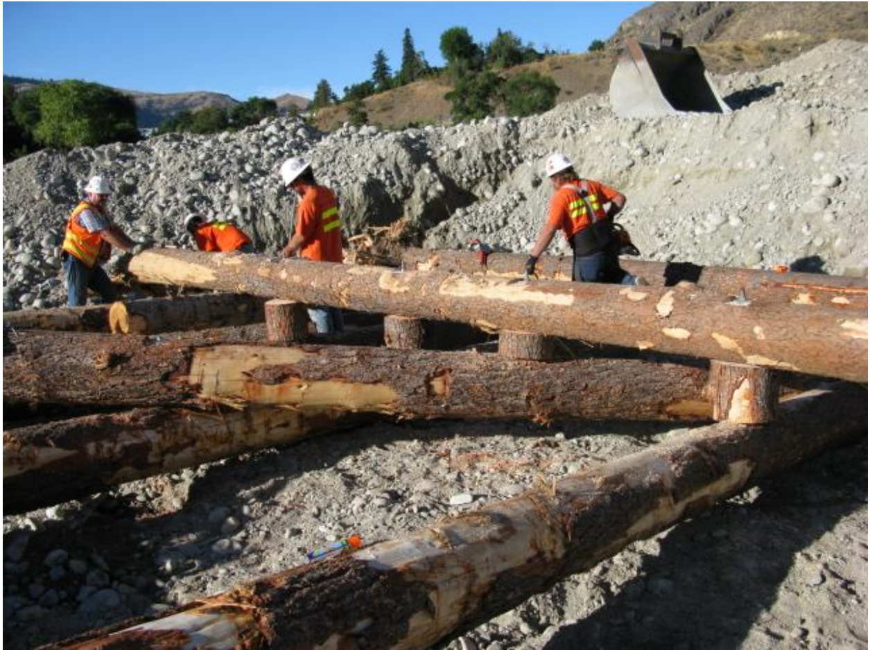
Construction of a log-jam rack. Includes shimming and bolting units together. August 29 th , 2008.
