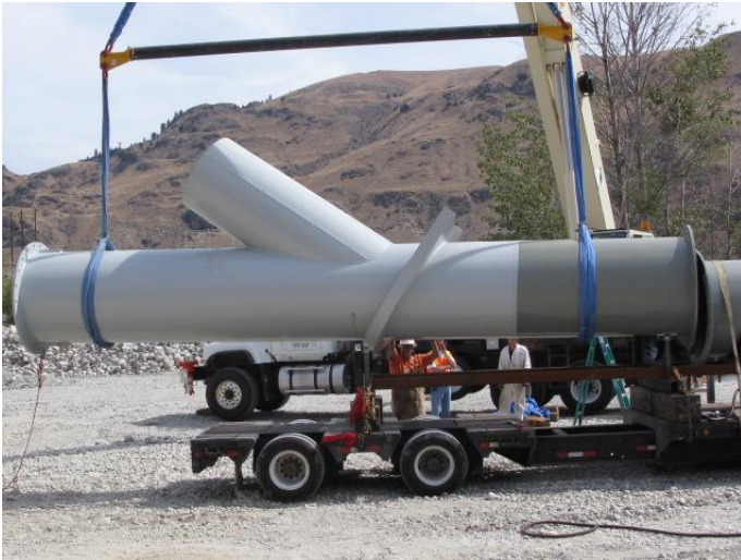
Receiving the pump tubes for the pumps. September 2 nd , 2008.
