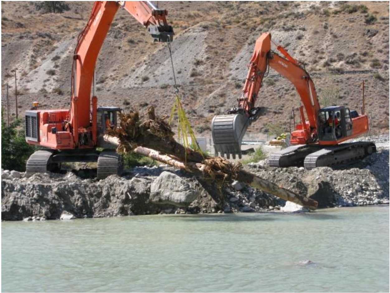
Setting a V-log jam in the lower Habitat Channel, in the water. August 27 th , 2008.
