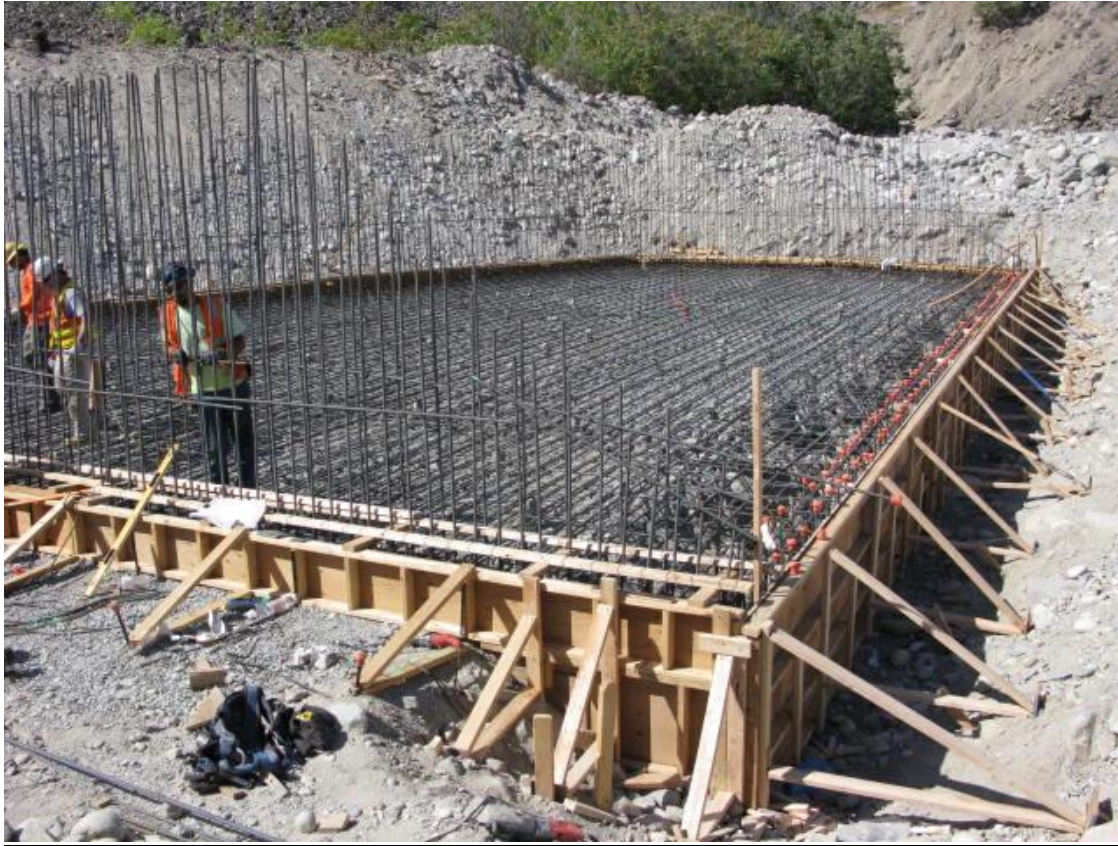
Pumped water outlet structure slab forming and rebar installation. This is a scheduled 170 cy concrete placement. August 21 st , 2008.
